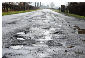
Figure 4.1: Damaged road surface
